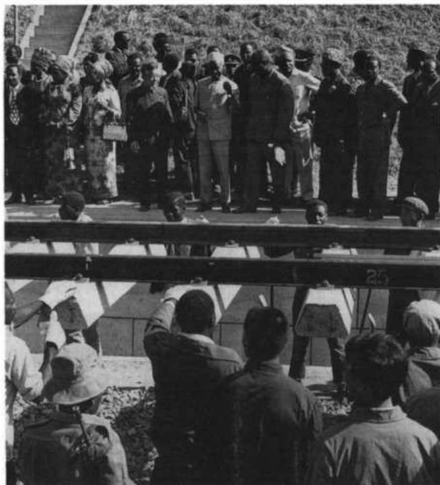
PLATE 27.3 The Chinese-built 'Green Uhuru Railway', Tanzania-Zambia: the laying of the track across the Tanzania-Zambia border, September 1973, in the presence of Chinese officials and Presidents J. Nyerere of Tanzania and K. Kaunda of Zambia
